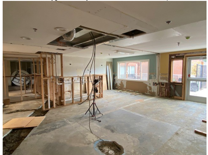
Above and below-plumbing and electrical rerouted and walls removed and reframed with steel beams to create spacious classrooms
